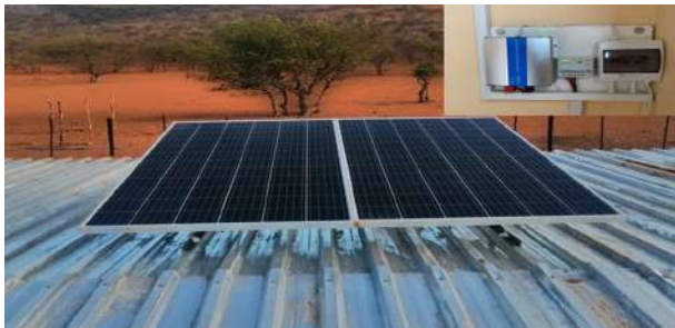
A Solar Home System typically has the capacity to power lights and devices such as radios, TVs, fridges and cell phone chargers.
